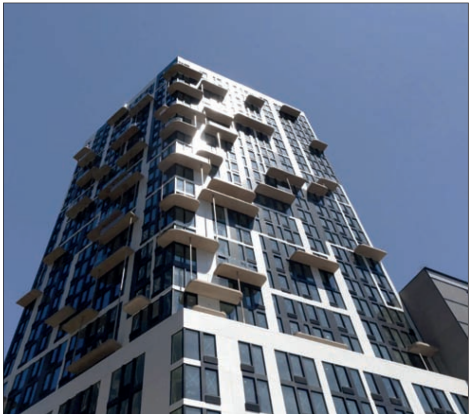
A residential development took shape along Flatbush Avenue in Brooklyn, May 1, 2026.
